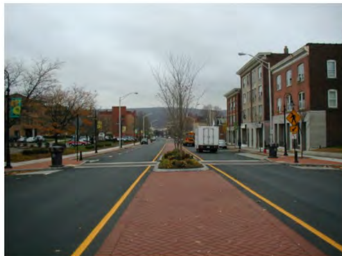
RAISED CONTRASTING PAVEMENT
