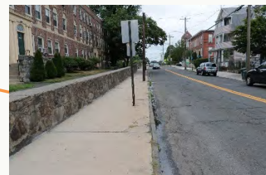
Protect existing stone wall, limited sidewalk width
