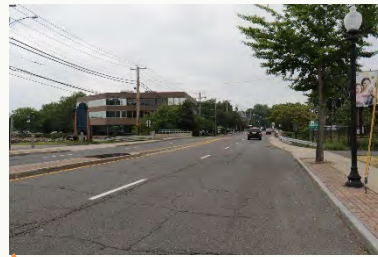
Street trees missing from median, decorative lighting and pavers need refurbishment
