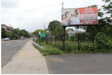
Billboard, overgrown vegetation and chain link fence at top of creek bank
