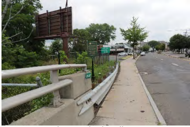
Roadway and sidewalk narrows at bridge
