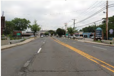
Expansive pavement, overhead powerlines, poor condition of pavement, lack of street trees
