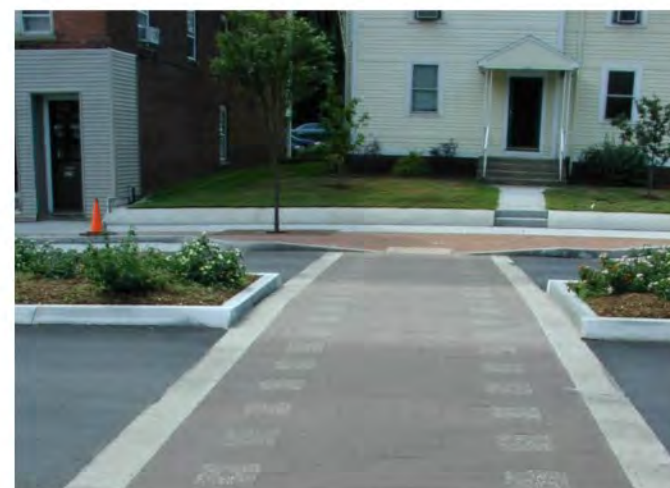
CROSSWALK— ASPHALT PAVERS
