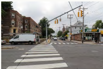
Very wide roadway, long distance for pedestrians to cross, lack of street trees
